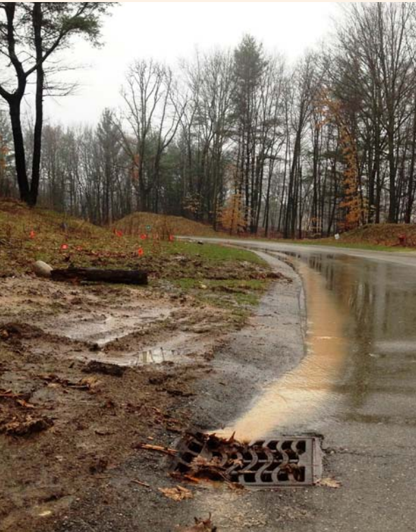
Polluted stormwater runoff is a common problem from construction sites and parking lots.
